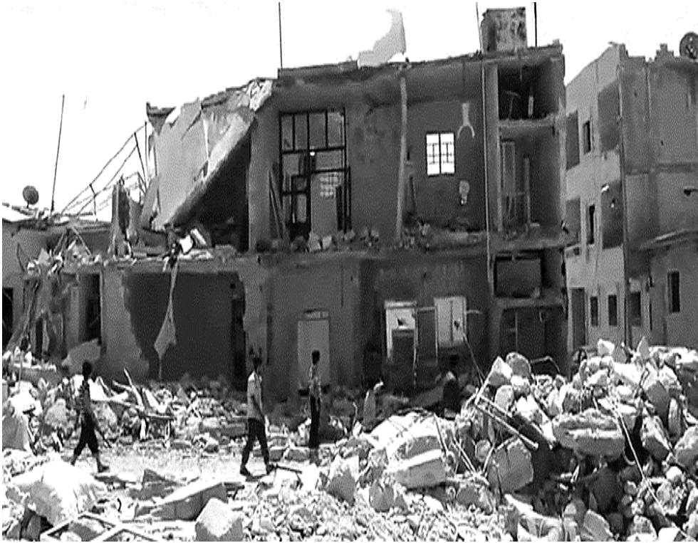
Figure 1. Destroyed place in Syria [23]
